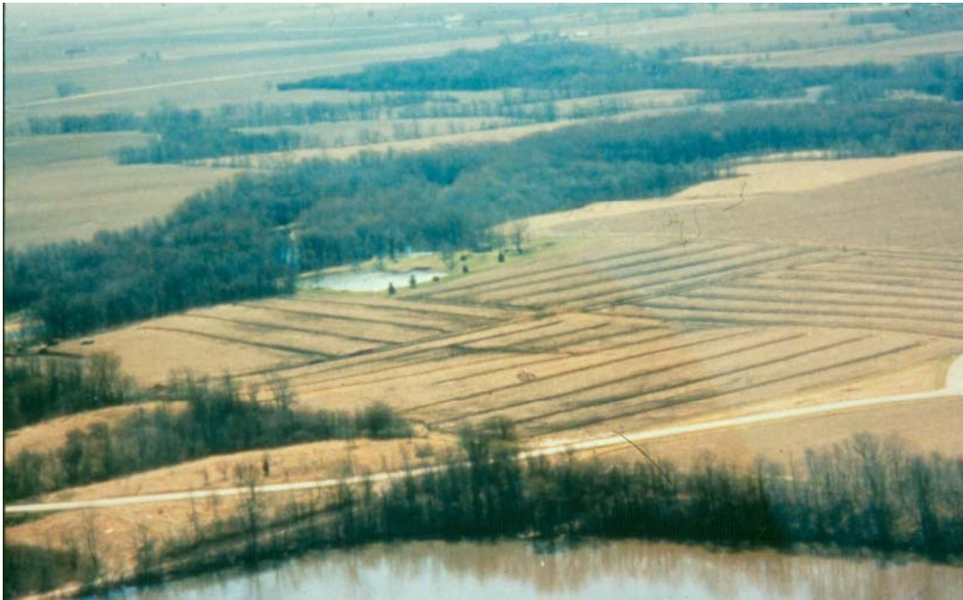
Figure 12. Aerial view of the tile site shortly after tile installation in 1997. The individual tile drainage networks for the six 5 acre treatment plots can be seen. This view is to the southwest, with the farm pond in the background. The wetlands were later built on City property adjoining the field at the left side of the photo.
