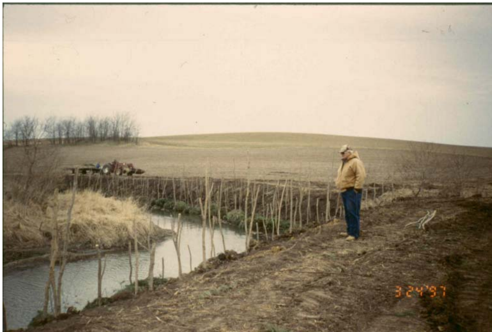
Figure 14. Dormant willow posts after installation.
